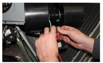
Connect jumper harness wiring harness
