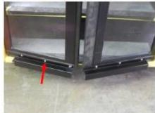
b) Using a Phillips screwdriver, remove both screws (up and down) on the door frame, which are holding the seals in place.
