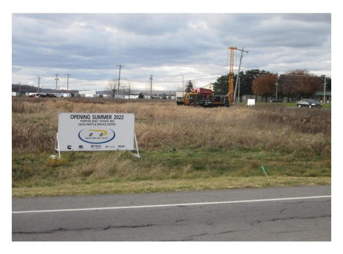
A drilling rig is currently on site to obtain soil samples to ensure compaction is sufficient for the foundation for the planned 20,000 square foot facility which will feature 11 Service Bays, parking for 150 buses and EV charging stations. Plans call for the facility to be fully operational in the second half of 2022.
